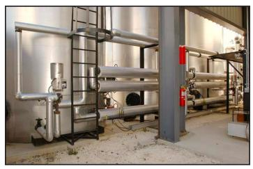
Astec normally pre-pipes the blending system at our factory using jigs for critical fits. This significantly reduces piping errors, speeds up field installation and reduces field re-works.
