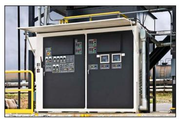
The main control panel for an early Heatec polymer system at an asphalt terminal. The operator initiates the blending process using controls on this panel. A PLC in the panel sequences the operations. Fiber-optic wiring, which is not affected by lightening strikes, can be used to interconnect panels in the system. Some of the controls on this panel are now replaced by a conventional desktop computer like the one shown above.
