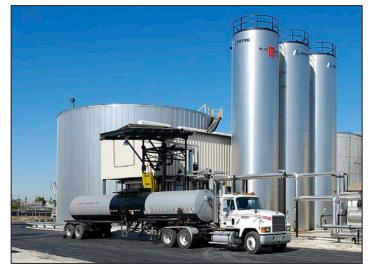
The three vertical tanks shown here are for polymer-asphalt storage. They are heated, insulated, and have mixers. Each tank holds 35,000 gallons.
