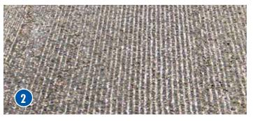
Standard <sup>5</sup>/<sub>8</sub> inch (16 mm) Single Hit Triple Wrap - 100 FPM
